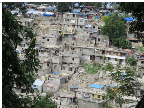
Earthquake damage in Haiti
