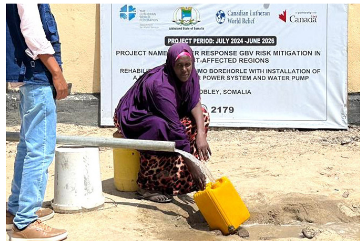
Ebla tests the pump of the newly rehabilitated solar-powered water borehole. (LWF photo)
